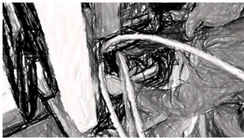
Image: Fastening the cables with the cable clamps
