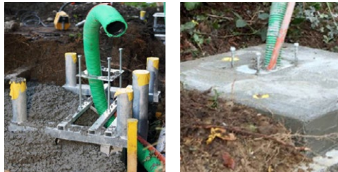
Pictures: concreting and laying the foundation
