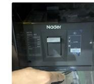
2. The circuit breaker trips and switches off
