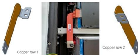
Take the copper busbar 2 (1x), hexagon head screw M6 (2x), flange nut M8 (1x) from the accessories. The second and third groups of battery modules are fastened on the right with the copper busbar 2 and tightened with a socket spanner. Check the tightening torque with a torque spanner (10 Nm for the M6 screw, 15 Nm for the M8 flange nut) and wrap the assembled unit with high-temperature insulating tape. Close the top and bottom flaps of the battery compartment and tighten the screws.
